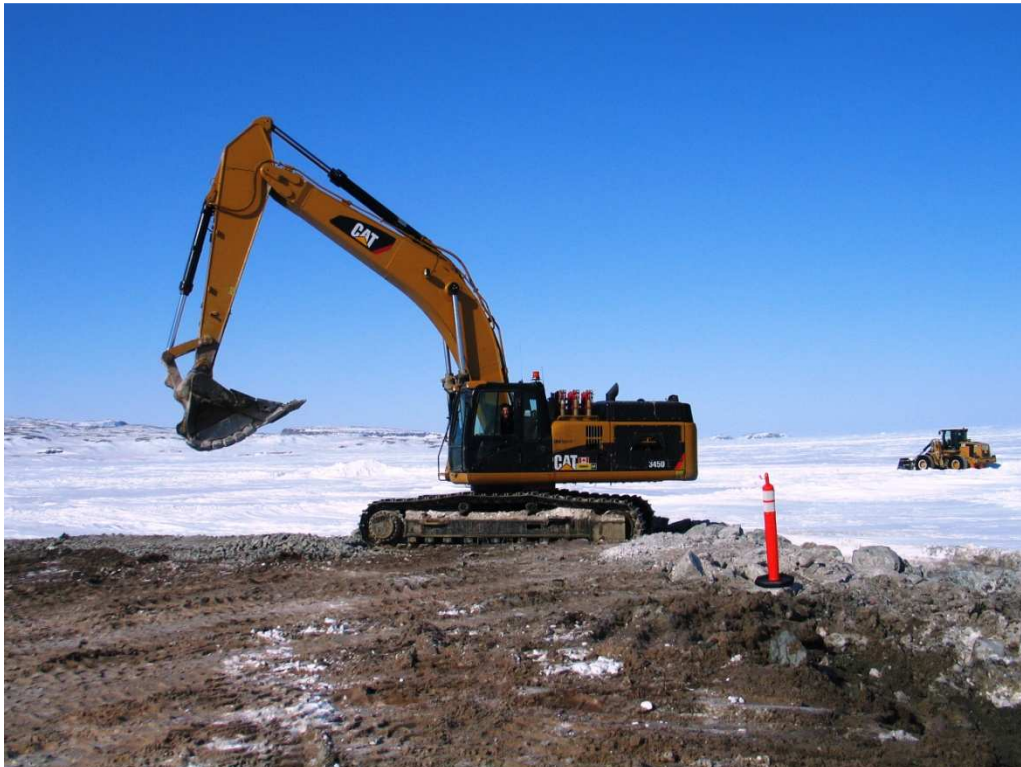
PHOTO 3: Excavator placing rip rap at the jetty.
